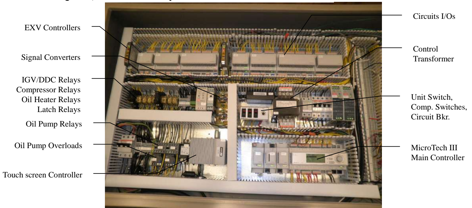
Figure 6, Control Panel Layout
